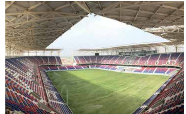
Iraq Stadium Roof Truss 650 Ton
