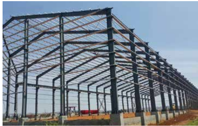
Uganda Steel Structure Warehouse 3830 m 2
